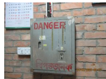
Electric Sub Distribution Box.JPG
