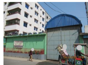
The facility used the front road as fire assembly point which is excluding existing risk assessment. (2).JPG
