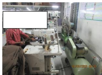
compressor machine found without safety barrier in production floor.JPG
